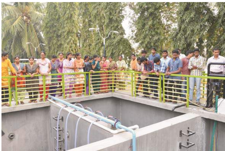
Moving Bed Biofilm Reactor
