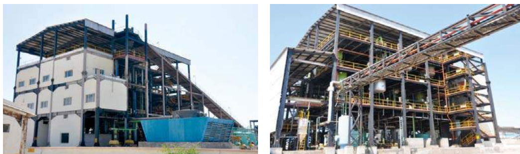
Sulphate of Potash Plant view
