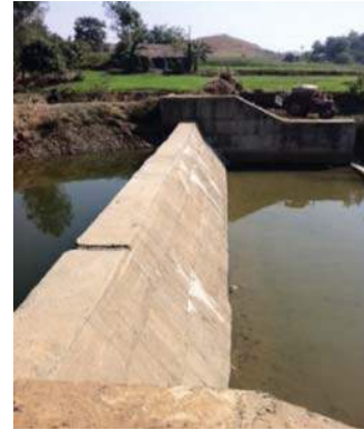
Check Dams and Catchment areas for Ground Water Recharge in Sabarkantha District, Gujarat
