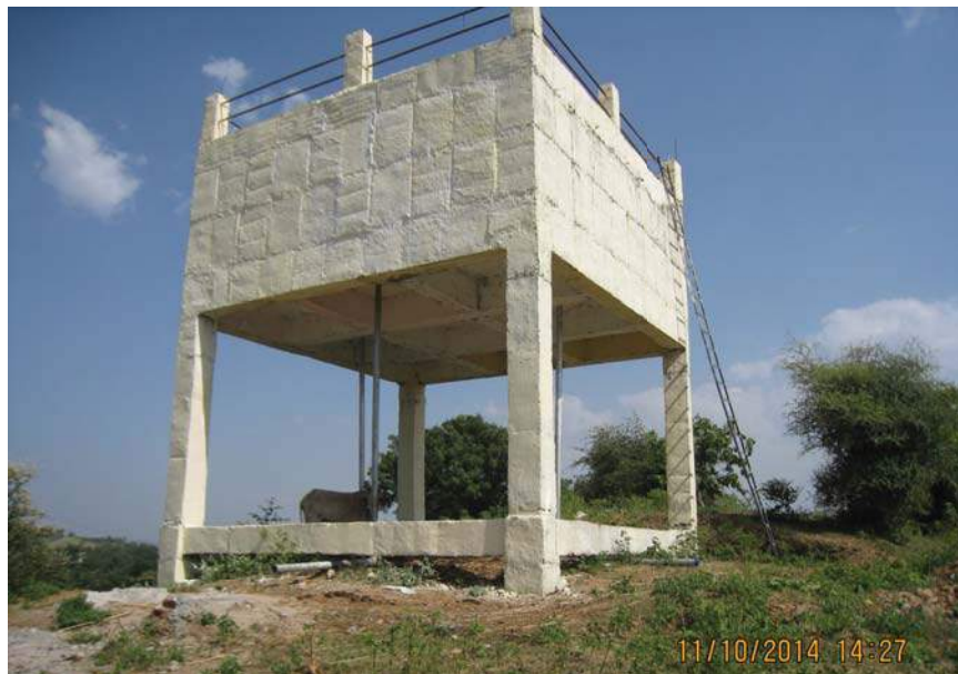
Overhead Community Reservoir in Sabarkantha District, Gujarat
