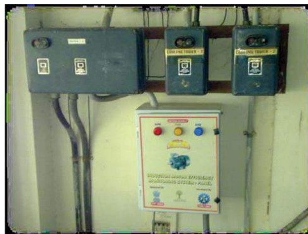
View of the Power Interfacing Unit fabricated & installed at Site
