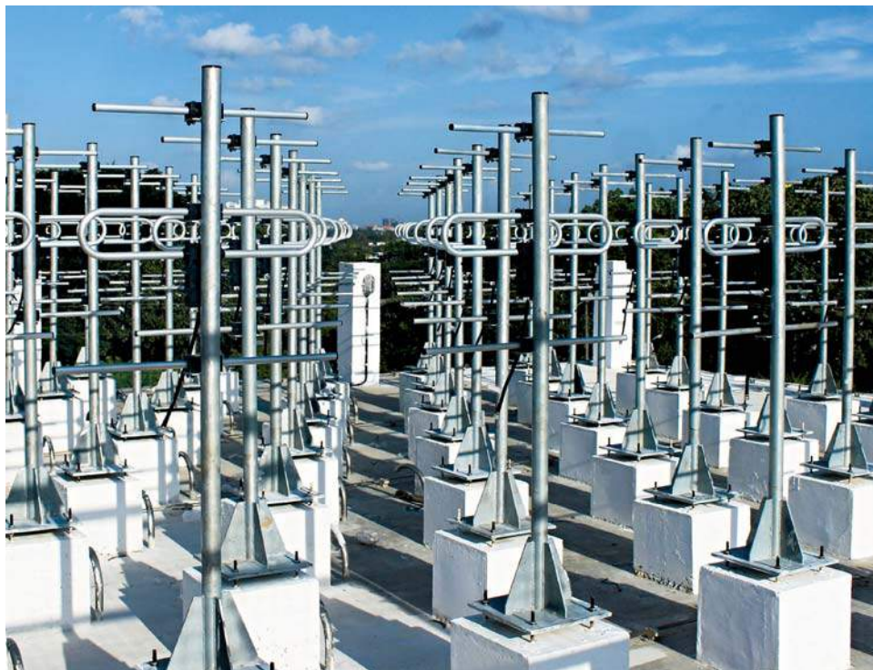
Figure-5: A Prototype 49-element antenna sub-array of ST Radar developed at CUSAT, Kochi
