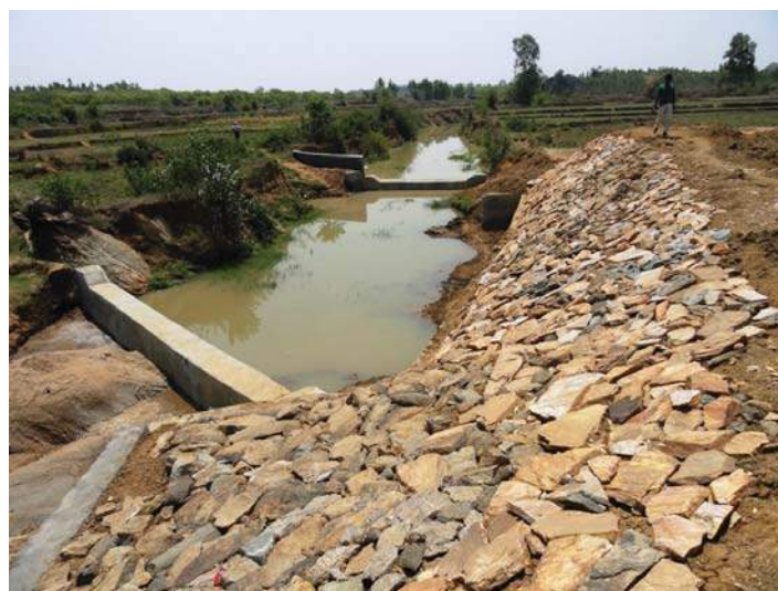
Check dams for ground water recharge
