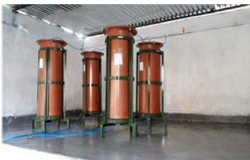
Low cost Laterite Arsenic Filter (Left) and Arsenic filter at Chouduar Primary School in Malda District, West Bengal
