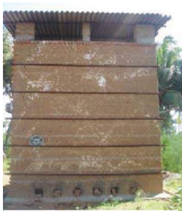
Modified Brick Kilns
