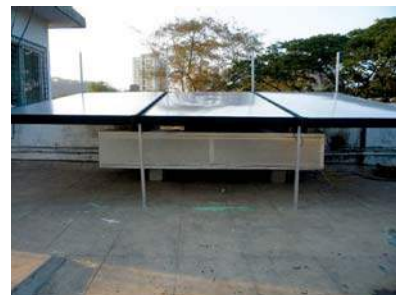
Solar Aluminium Tubular Air Heater developed by IIT Bombay
